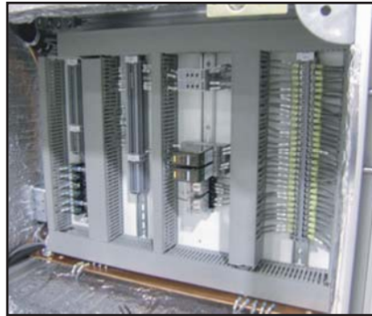
Low voltage control compartment
